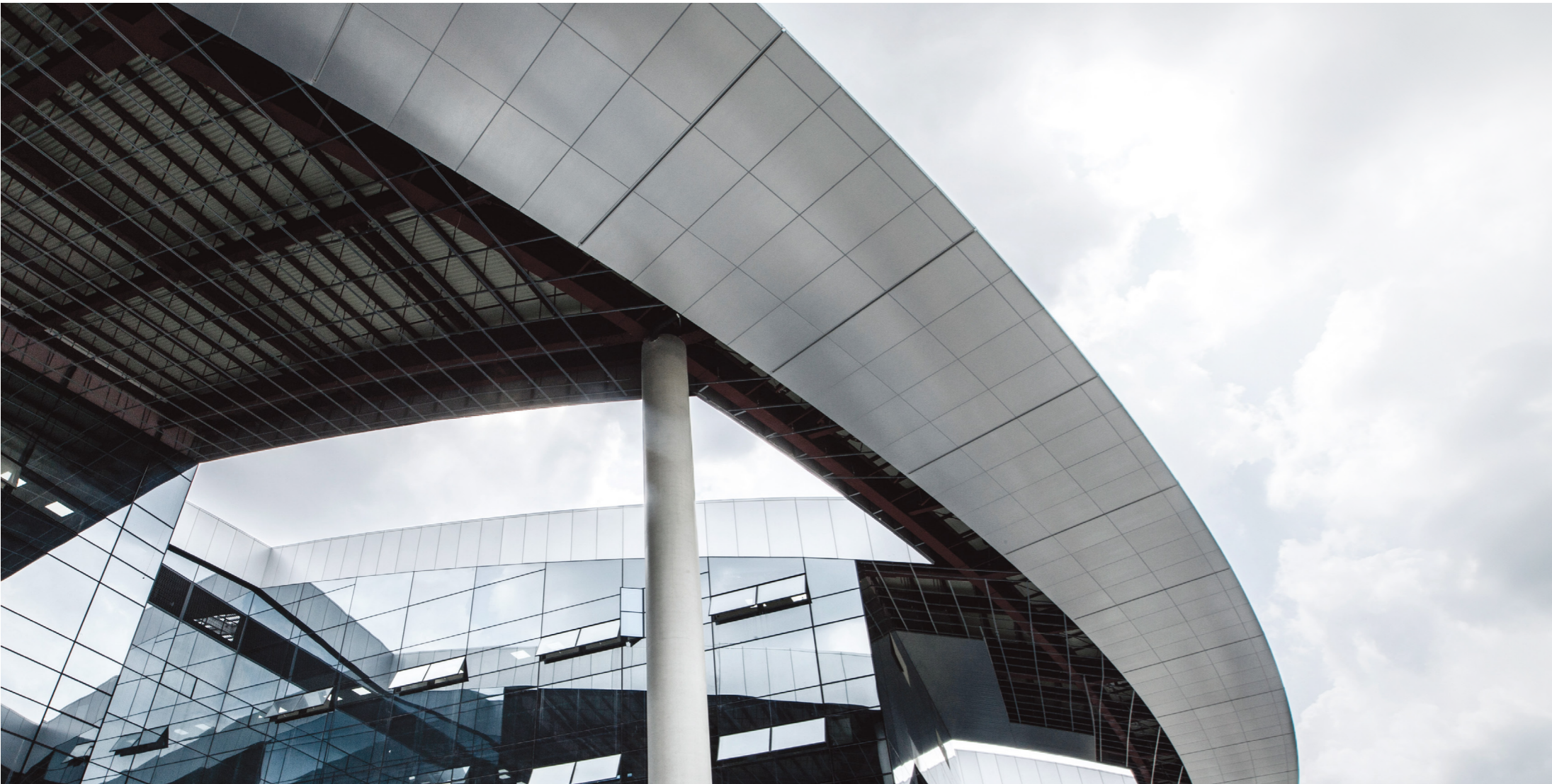
Exterior of Hankook Technodome
